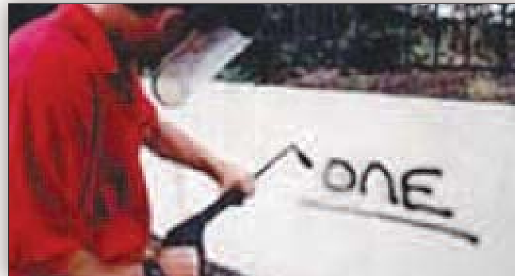
Graffiti cleaning contractor
